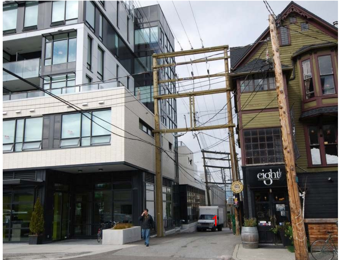
View down the side service lane that gives access to the basement parking garage.
